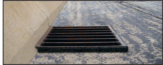
Steel risers are typically installed just before final paving lifts, as in this I-39 example.
