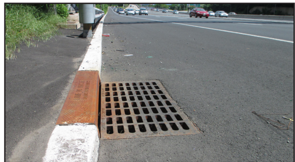
On Route 78, 450 catch basins ended up perfectly flush with new paving.
