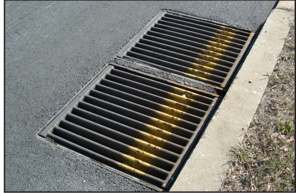
Because they are customizable in fine increments, steel risers leave inlets and catch basin grates precisely at grade.
