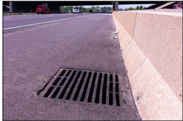
On this I-64/I-255 resurfacing project, the project engineer estimated that use of 100 steel risers saved nearly two weeks of construction time.
