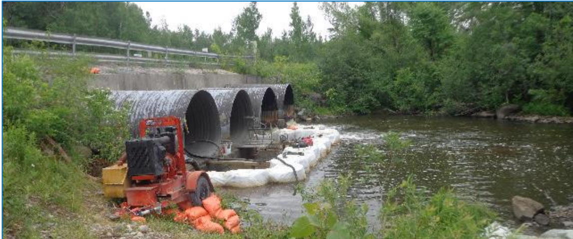
Figure 3: Parallel 142” by 91” CMP Road-Supporting Arches, Fort Drum, NY
