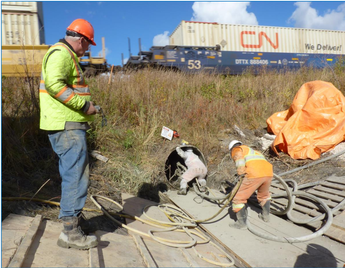
Figure 11: Rehabilitating under active rail lines in remote areas
