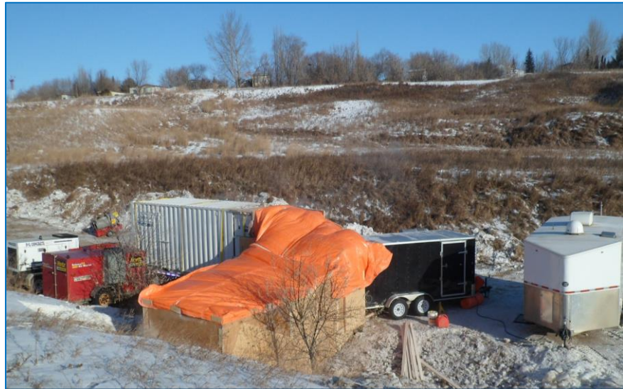
Figure 12: Enclosed, heated work space
