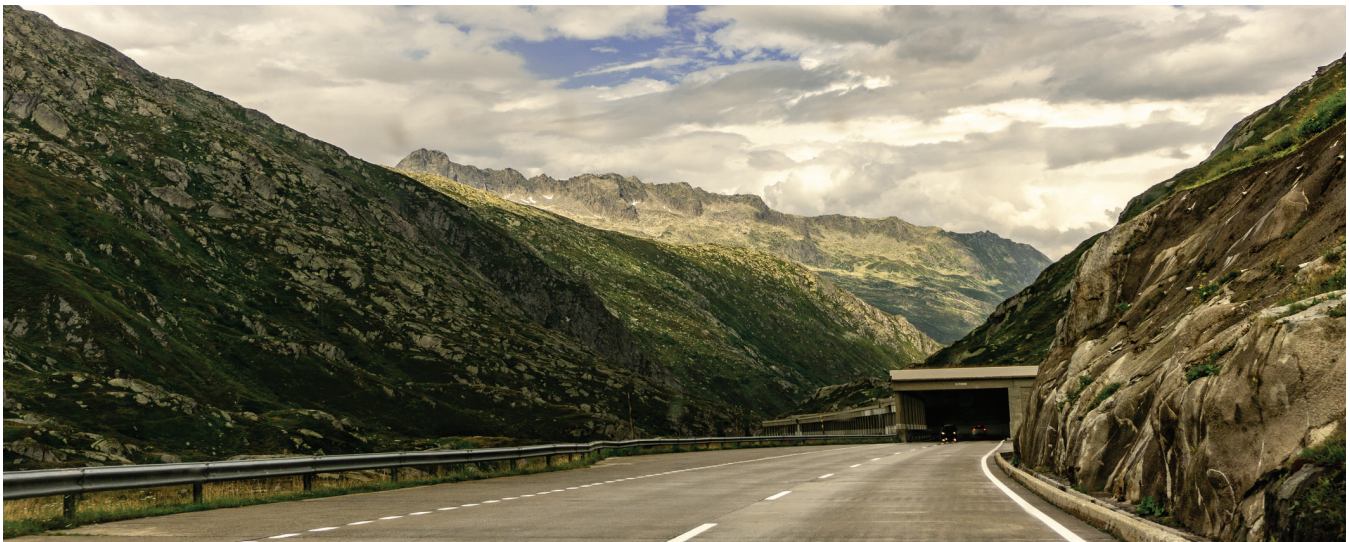
The Gotthard Base Tunnel, running deep under the Swiss Alps, is the longest railway tunnel in the world, at just over 35 miles in length. Because of the project's complexity, construction teams often worked simultaneously on different sections of the tunnel.
