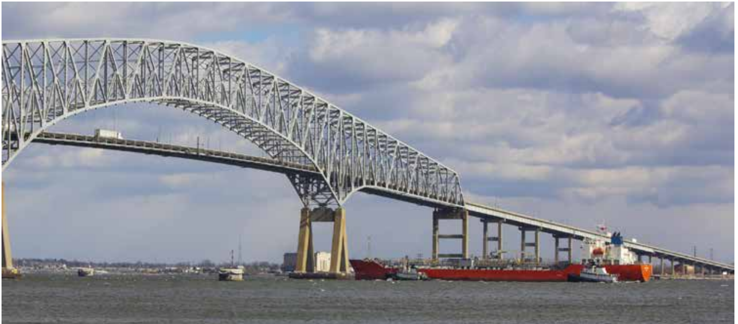
Photo of Francis Scott Key bridge in Baltimore.
